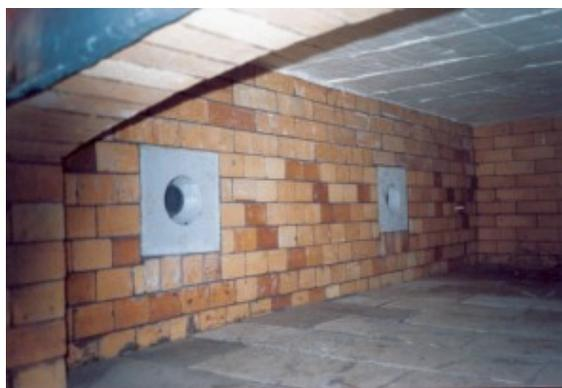
**Figure 2b. Refractory walls of a furnace interior with burner blocks** (BEE, 2005)
